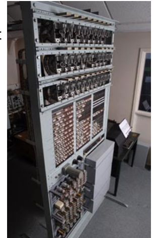
Tunny rebuild nearing completion
